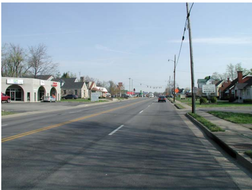
Figure 14: US 31E Northbound
